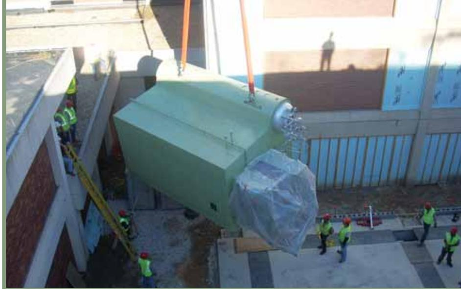
Among the biggest challenges for Great Baltimore Medical Center's boiler-replacement project was lack of direct of access to the work site on any side. To address the challenge, installers used a 650-ton crane to lower the boilers into place in the medical center's new plant.
