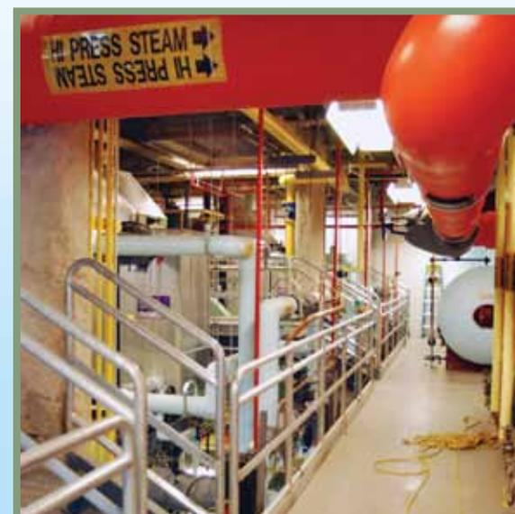
Greater Baltimore Medical Center selected three watertube steam boilers for its replacement project, which also included a new deaerator tank, a feedwater pump seat, and a condensate surge tank.
